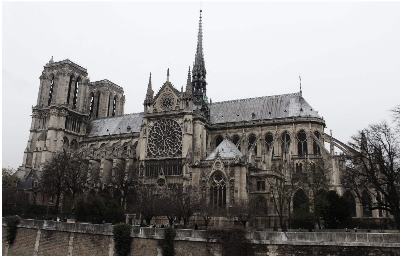
Figure 6 – South Elevation of Notre Dame, restored with fleche on central axis as seen today (Author's own)
