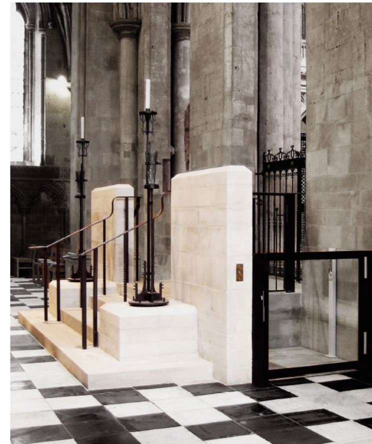
Figure 39 - Platform lift concealed behind steps into Shrine Chapel. ( http://www.rgarchitects.com/ )
